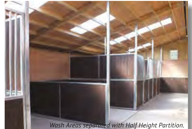
Wash Areas separated with Half Height Partition.
